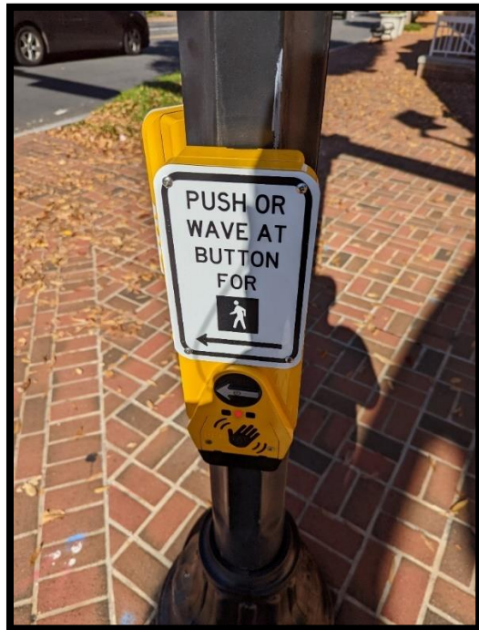
Figure 10: A crosswalk audio device present at the Chain Bridge Rd./North St. intersection
