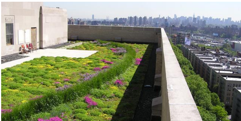
Figure 2: A typical intensive green roof with a mix of various sedum and grass species. Retrieved from https://greencitygrowers.com/blog/green-roofs-on-every-building/ .
