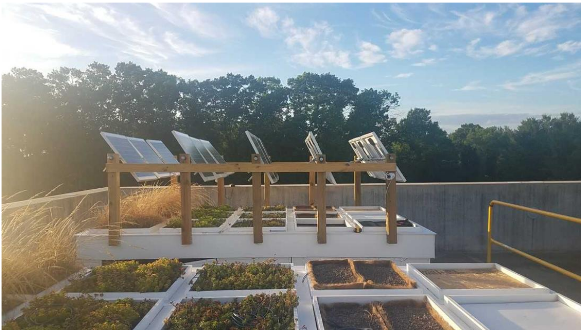
Figure 7: George Mason green roof installation during the Summer of 2017.
