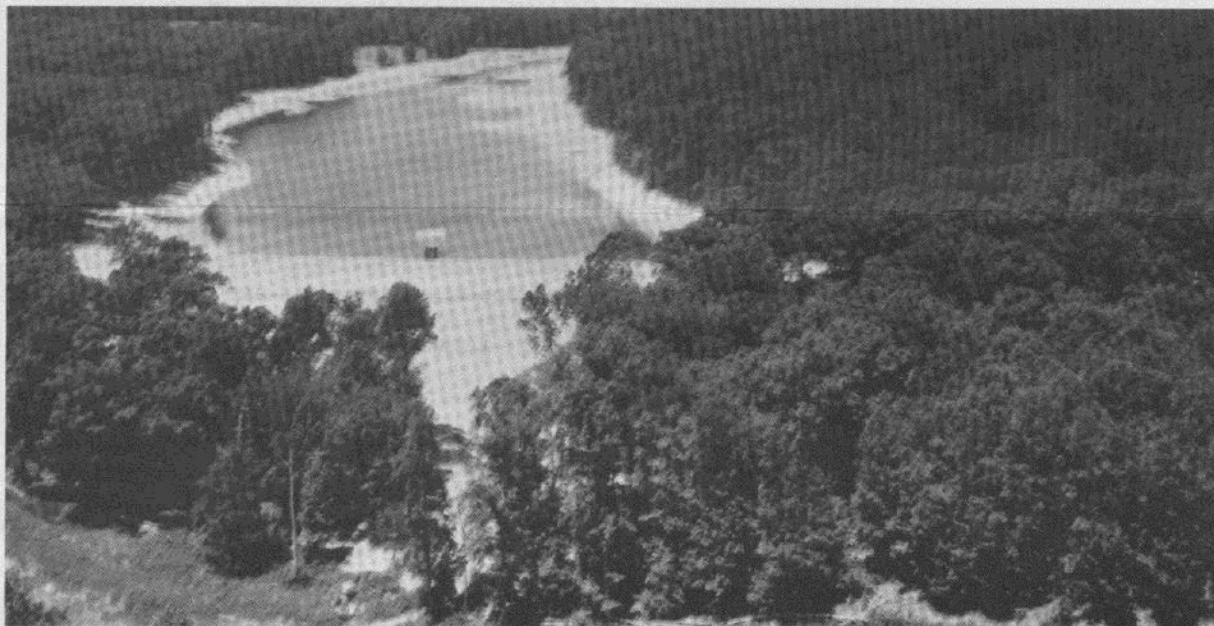
LAKE ANNE BECOMES REALITY: Aerial view shows completed dam and Lake Anne 30 percent full. Impounded water is used to irrigate 18-hole golf course. Lake is expected to be at full 30-acre level by mid-winter.
